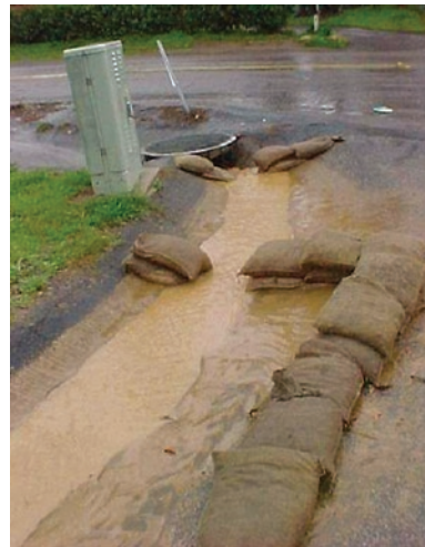
Figure 5. Make sure storm drain inlets are protected.
