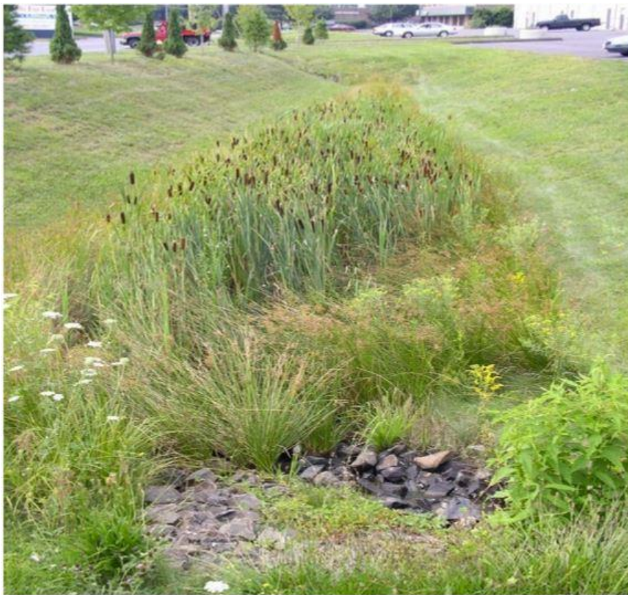
Photo 8. Example of a Wet Water Quality Swale from the CT Stormwater Quality Manual
