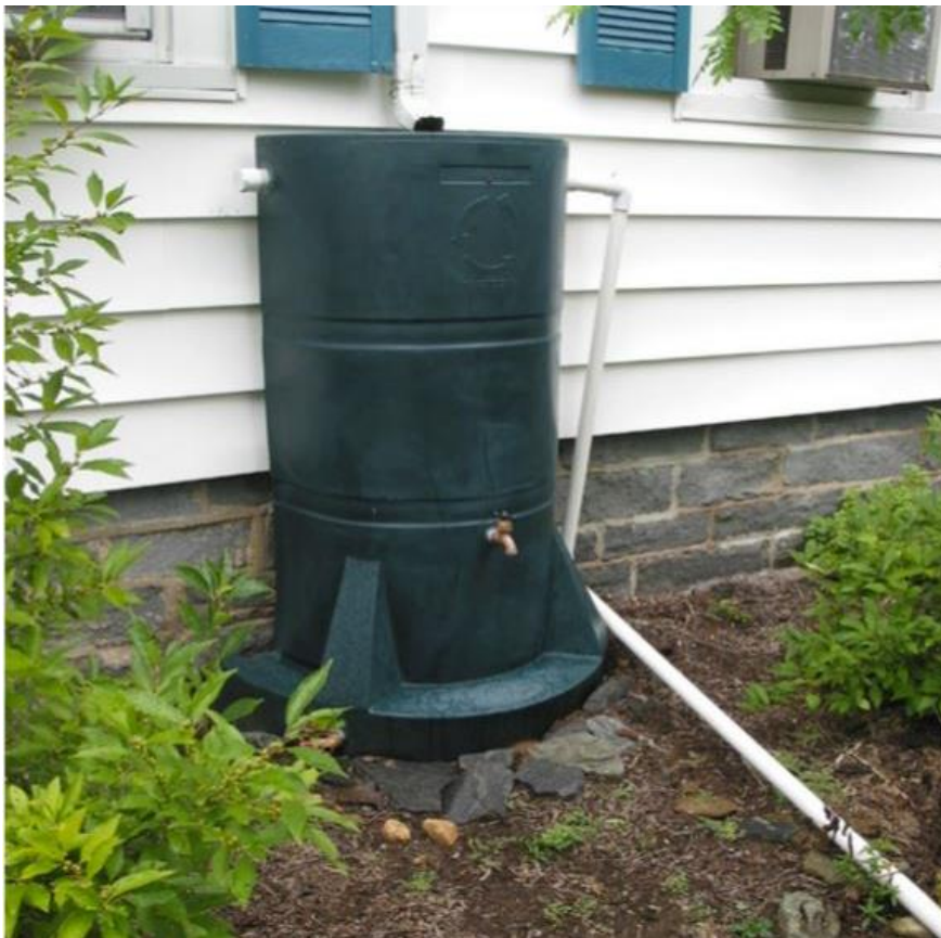
Photo 7. Example of a Rain Barrel from the CT Stormwater Quality Manual
