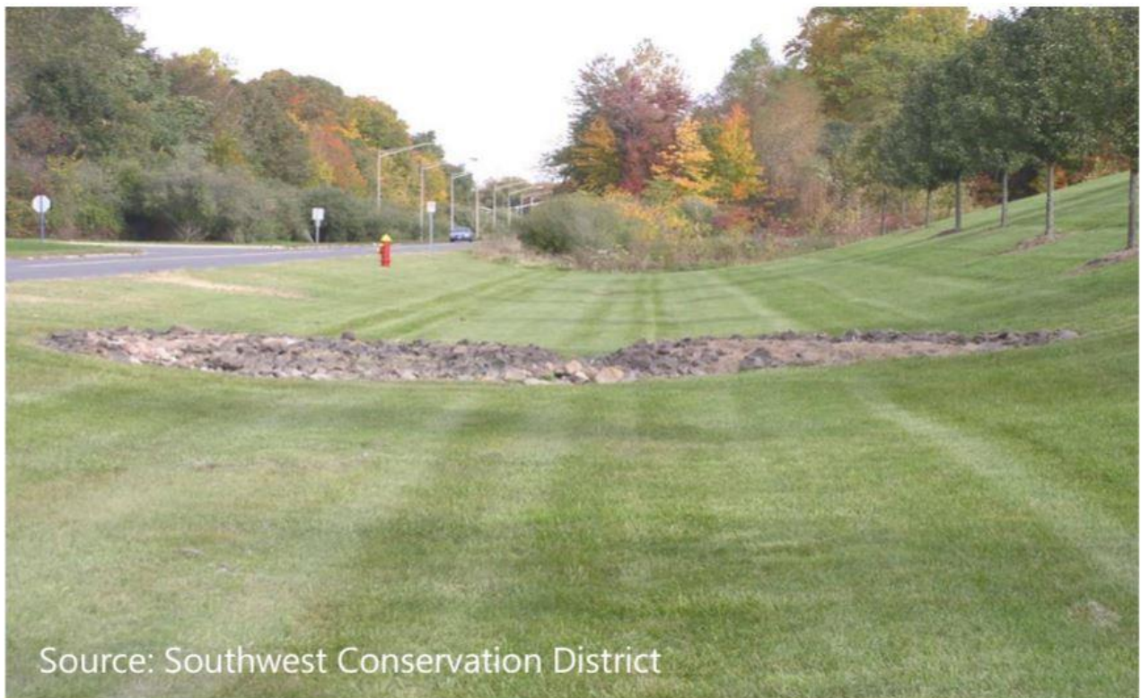
Photo 9. Example of a Dry Water Quality Swale from the CT Stormwater Quality Manual
